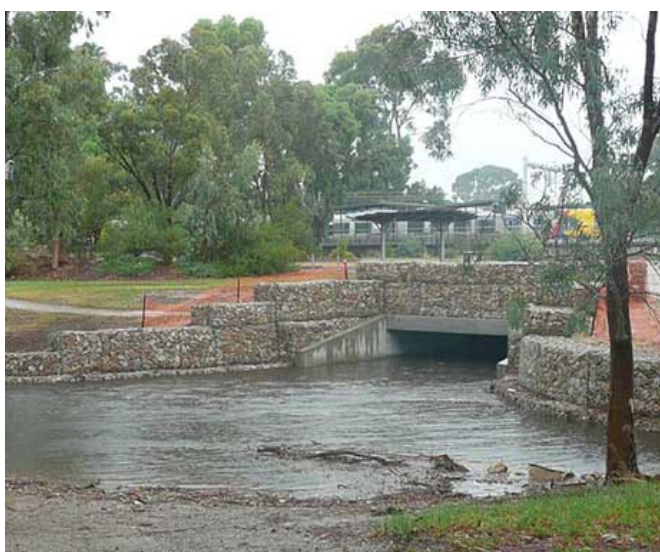
Constructed Culvert
