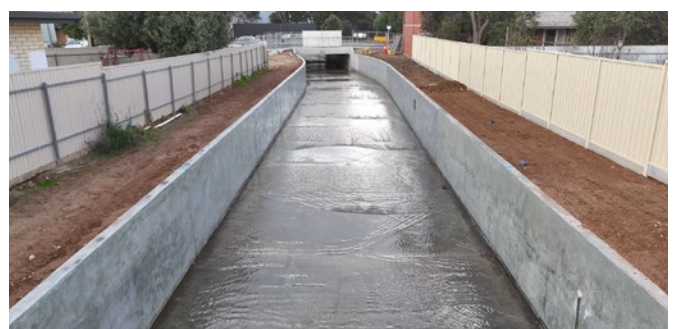
Channel construction through to completion
