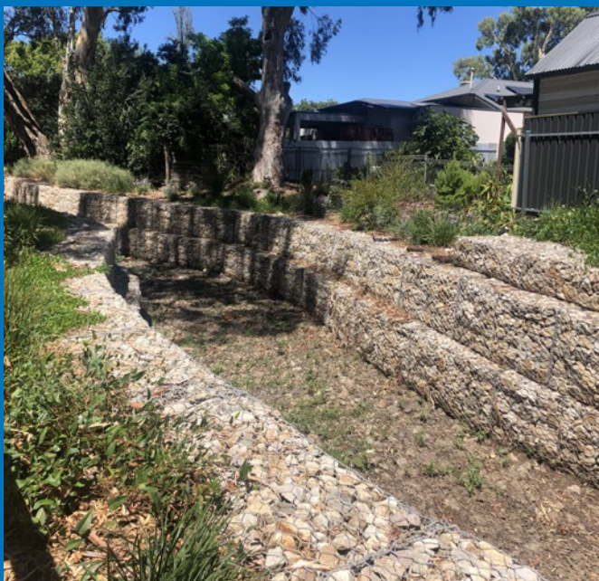
Rock filled gabions
