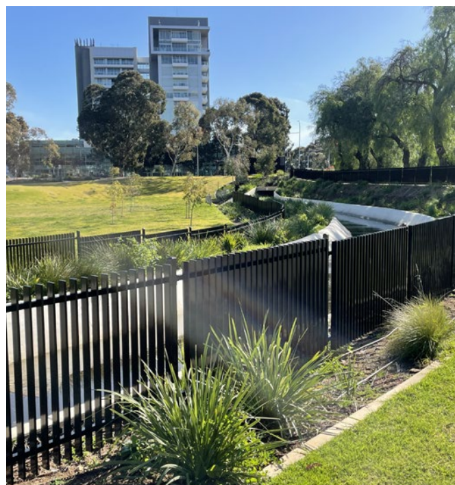
Concrete swale and fencing
